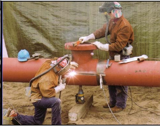
Fig. 2: Split-tee during welding. Photograph: Gasunie.
