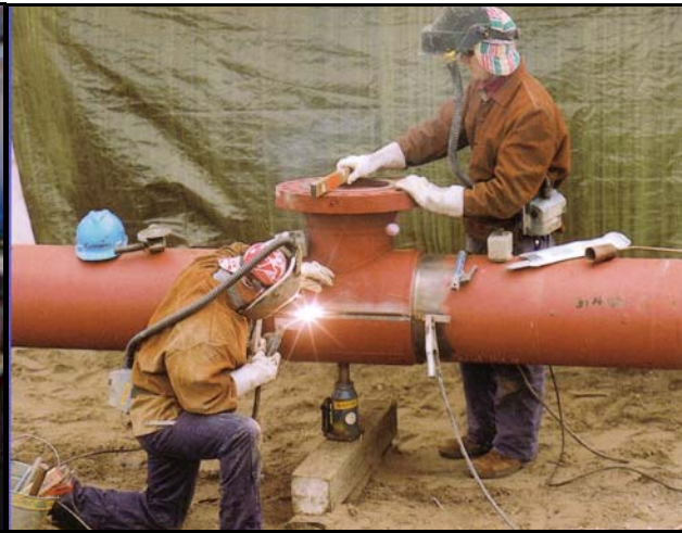
Fig. 2: Split-tee during welding. Photograph: Gasunie.
