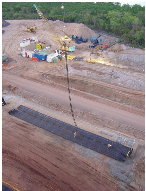
Figure 5 – Installation of prefabricated vertical tendons
