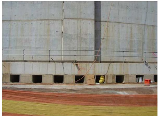
Figure 4 – Bottom anchorage recess for vertical tendons
