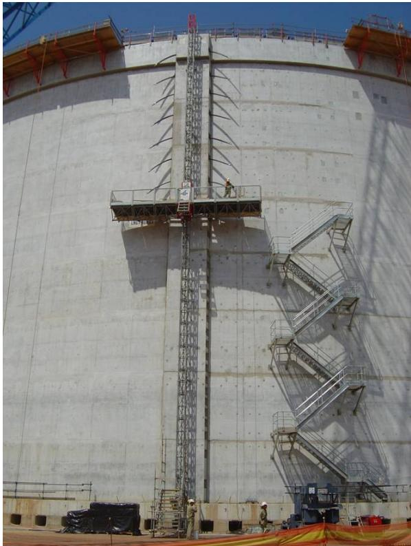
Figure 6 – Access platform at pilaster
