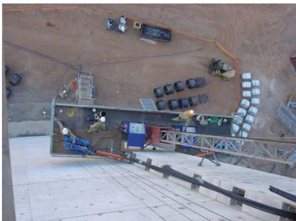
Figure 8 – Strand pusher operating on the access platform
