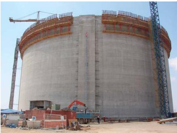
Figure 10 – 5<sup>th</sup> LNG Tank in Barcelona
