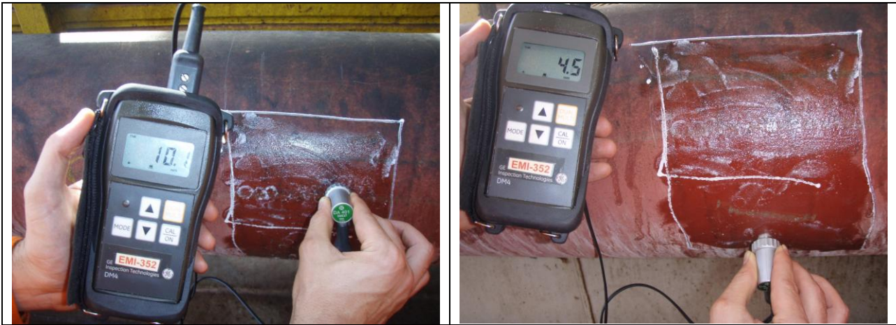
Figure 3. UT follow-up inspection on a 10” pipe schedule 40. On the left, thickness at the 3 o'clock position is 10.1mm. On the right, thickness at the 5 o'clock position is 4.5mm.
