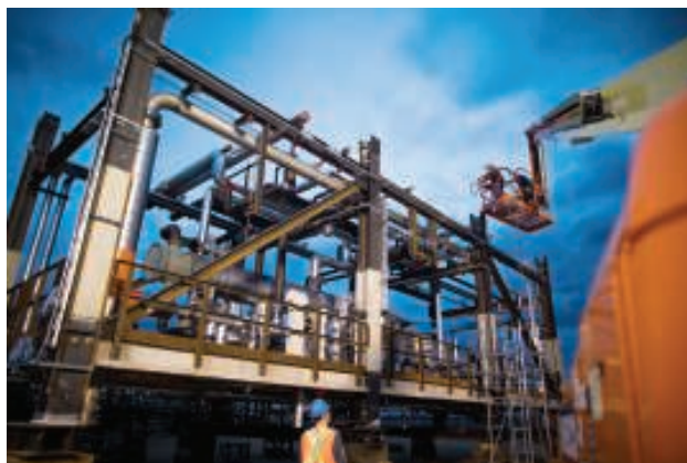
FIGURE 1. Modularization, the pre-assembly of structures away from the primary construction site, has many benefits, including improved labor productivity and reduced HSE risks
