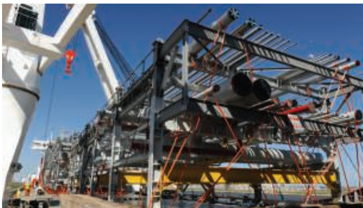
FIGURE 5. A module is prepared for transport to the project site
