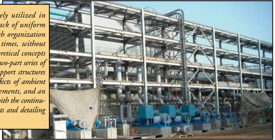
Side view of 4 tier process pipe rack with longitudinal bracing. Courtesy of Midrex Corporation, Inc., Charlotte, NC.
