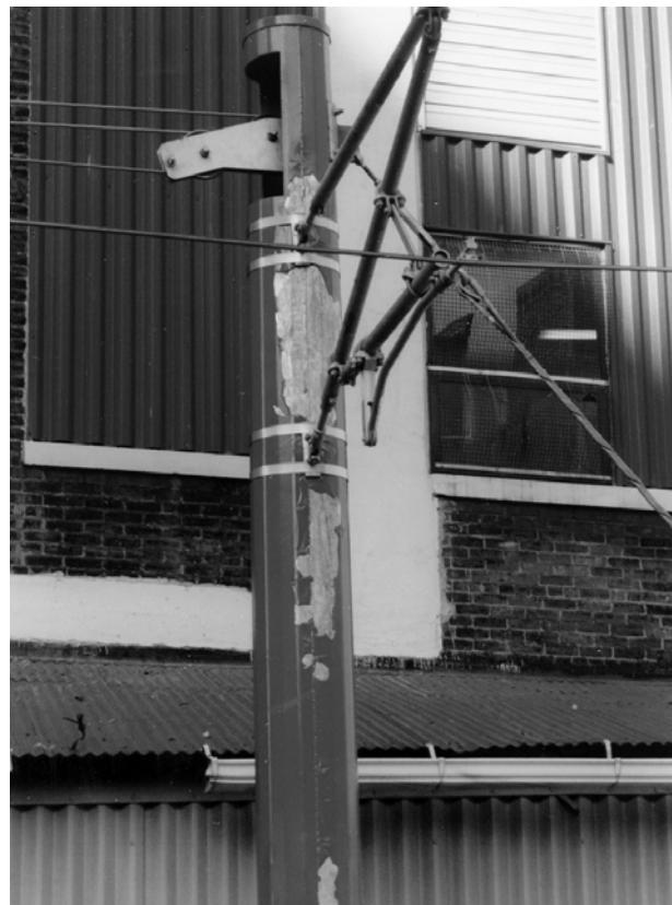
paint as a result of poor surface preparation. The surface contained zinc oxides and zinc hydroxides when the paint was applied. The coating appeared to adhere to the surface, but after two to three years in service, the zinc oxide began to separate from the underneath zinc metal. As paint was adhering to the zinc oxide, it separated from the pole surface at that time.
